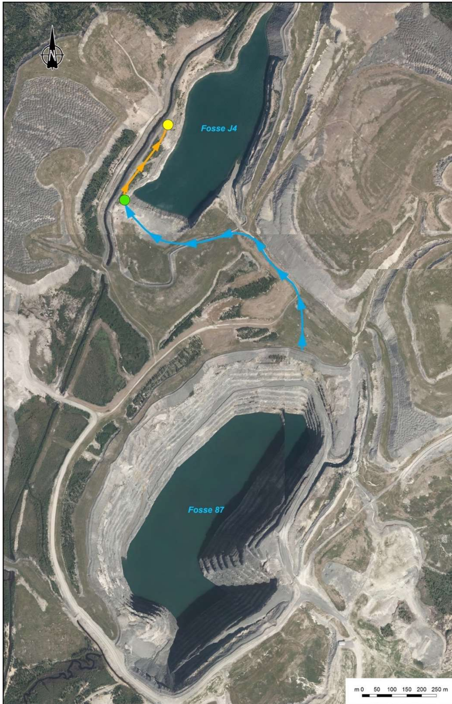
Figure 5.2 Water treatment plant location (green dot) and discharge point (yellow dot) and the discharge pipe from pit 87
