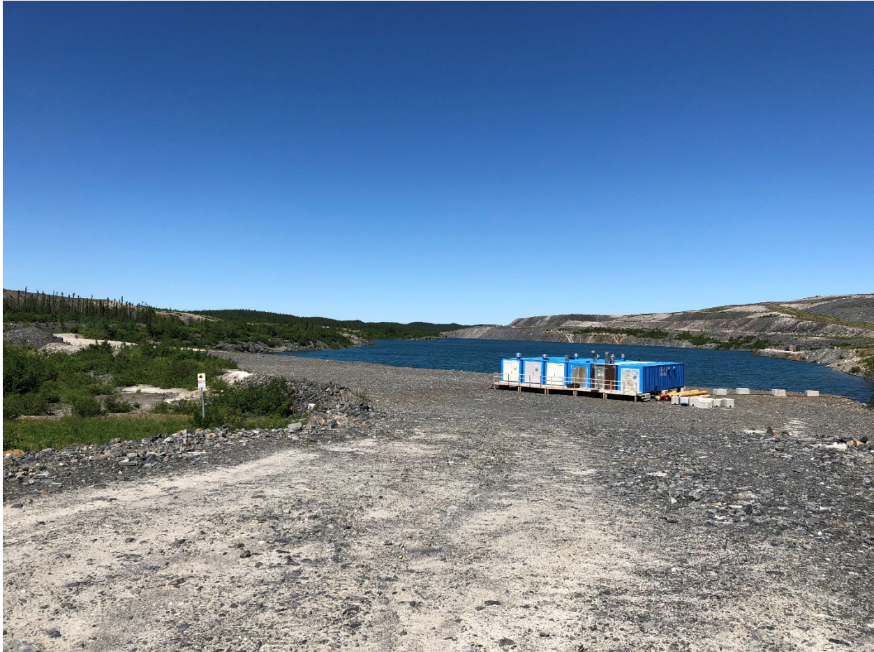
Figure 1: Water treatment and pumping facility at J4 pit
