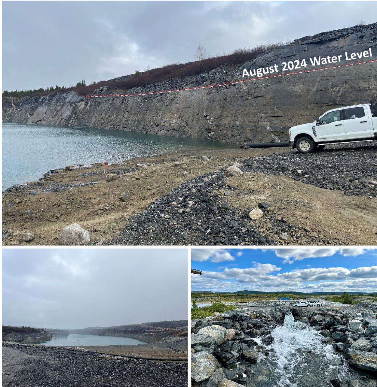
Figure 1. J4 Pit Dewatering Progress
