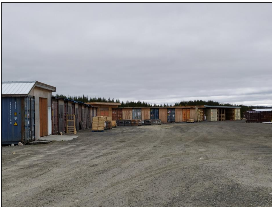
Figure 12-5: Core Storage Area; Pulp and Rejects Storage Facility
