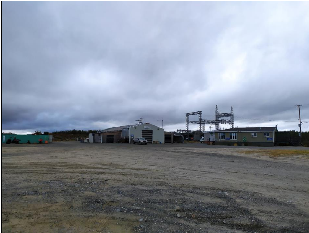
Figure 12-3: Core Logging Facility (centre) and Administrative Centre (right)
