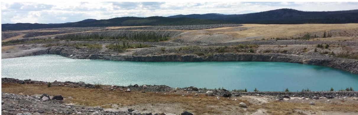
FIGURE 5-6 J4 PIT LOOKING SOUTHWEST AS OF JUNE 2016
