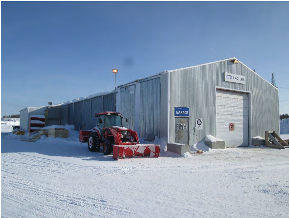
Figure 12-1: Drill Core Logging and Sampling Facility
